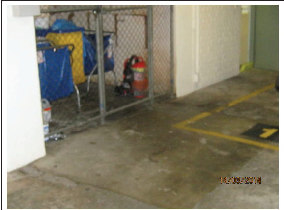
Photo 7: Location of UST in basement car park at 51 Pitt Street
