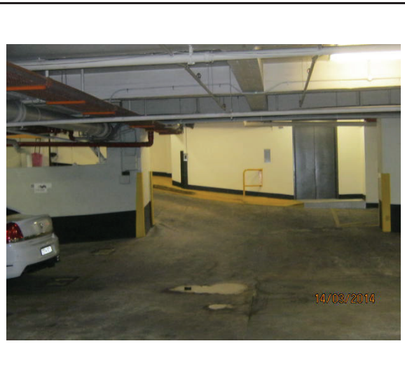
Photo 6: Entrance to car park at 51 Pitt Street
